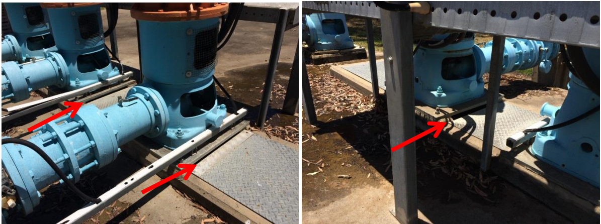
Figure 23 Vermin access points near distribution pumps
