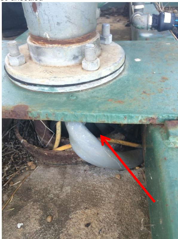
Figure 14 Active bore - also unsealed
