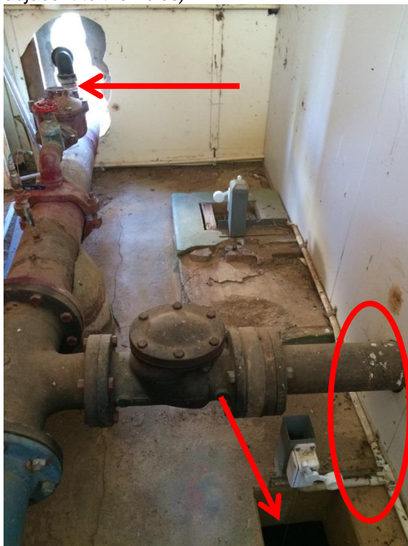
Figure 4 Further points of ingress into WTP building and into the clear water tank (under the floor)
