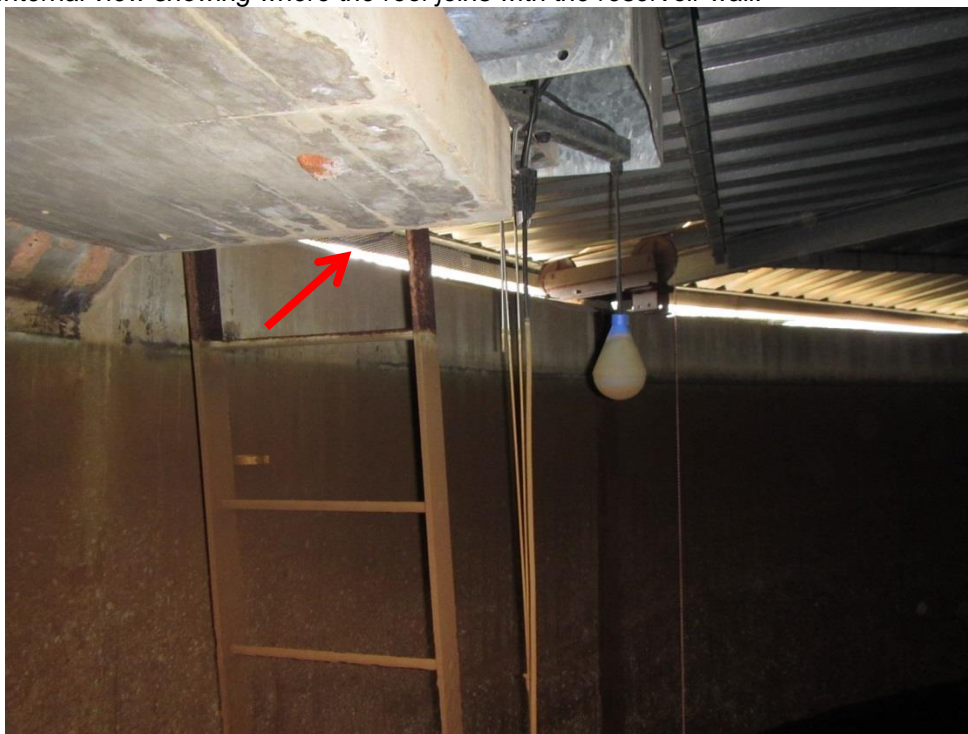
Figure 8 Internal view showing where the roof joins with the reservoir wall.
