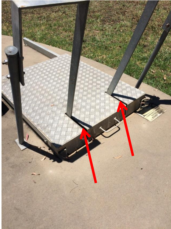
Figure 23 Vermin access points near distribution pumps
