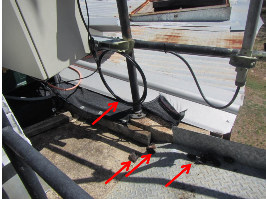
Figure 17 Martin St Reservoir - other points of ingress, and evidence of visible contamination
