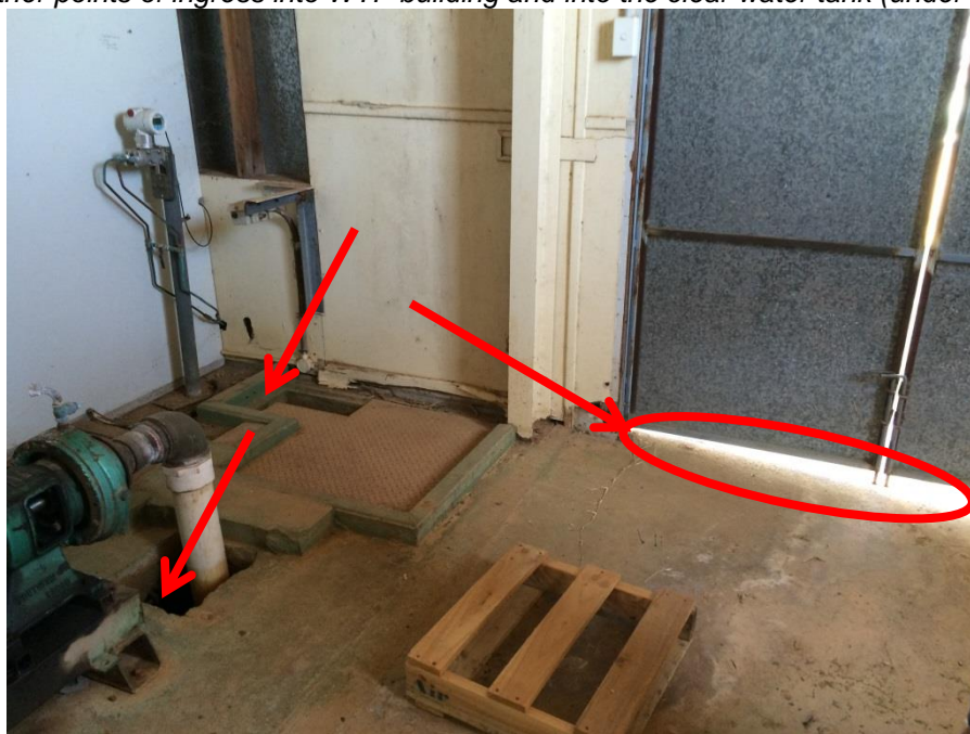
Figure 4 Further points of ingress into WTP building and into the clear water tank (under the floor)
