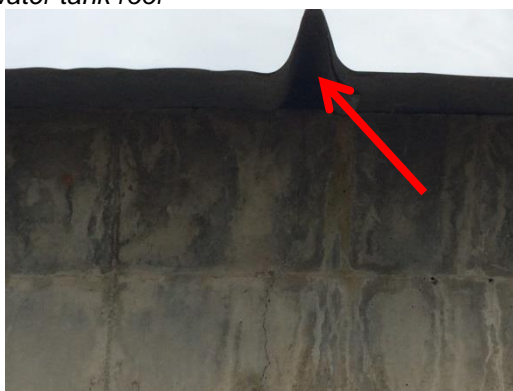
Figure 33 Mendooran clear water tank roof
