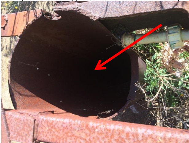
Figure 14 Active bore - also unsealed
