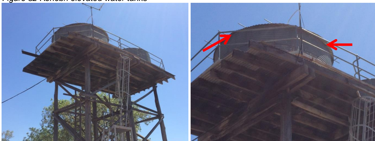
Figure 32 Kenebri elevated water tanks
