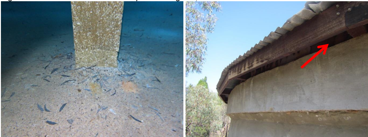
Figure 17 Martin St Reservoir - other points of ingress, and evidence of visible contamination
